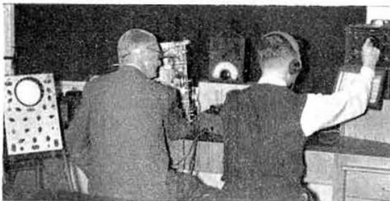
Lining up a crystal filter in one of the s.s.b. transmitters.
